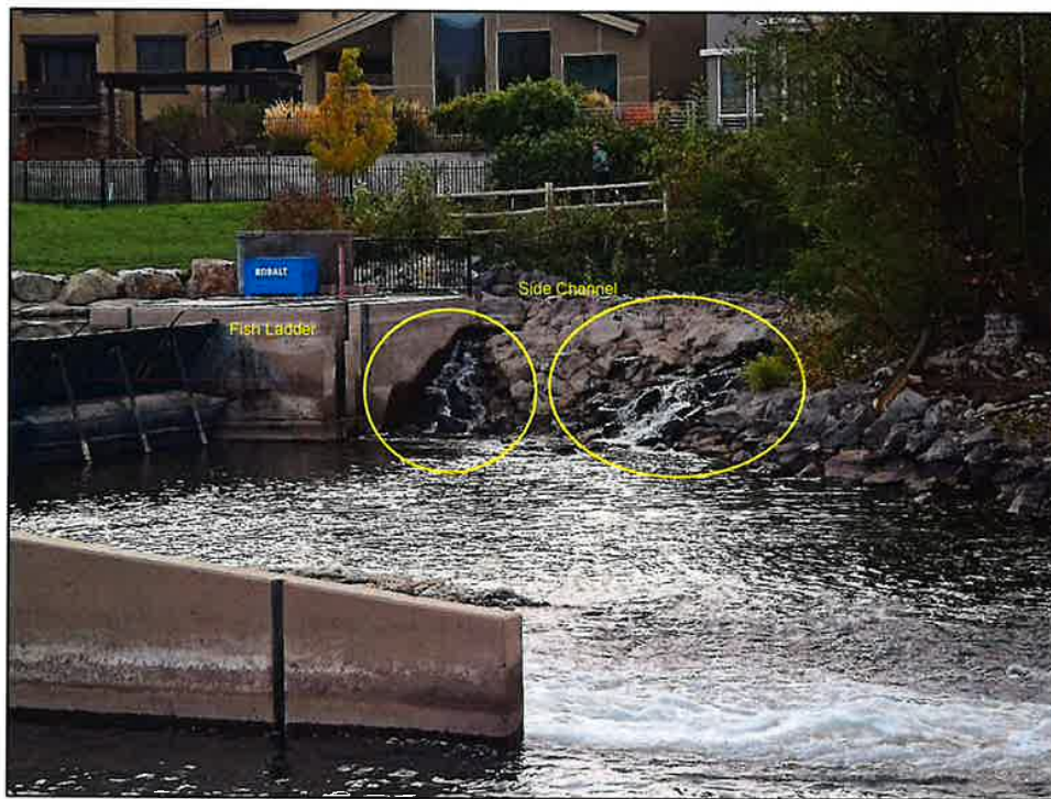
Photograph 4. Left Bank Side Channel Leakage Through Riprap and Grout (October 2023).
