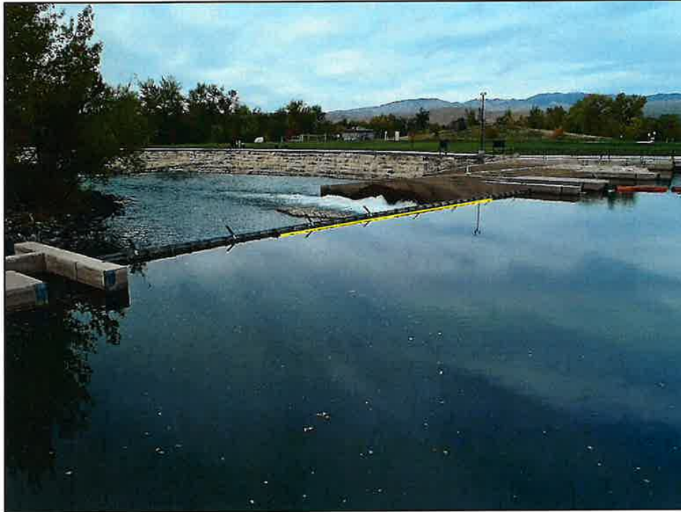
Photograph 1. Drop Structure 1 Gates 5 & 6 looking Downstream (October 2023).
