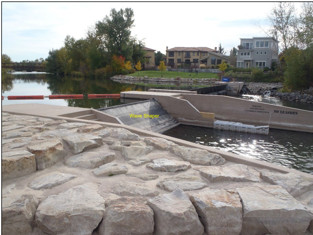
Photograph 5. Drop Structure 1 Wave Shaper looking Upstream (October 2023).
