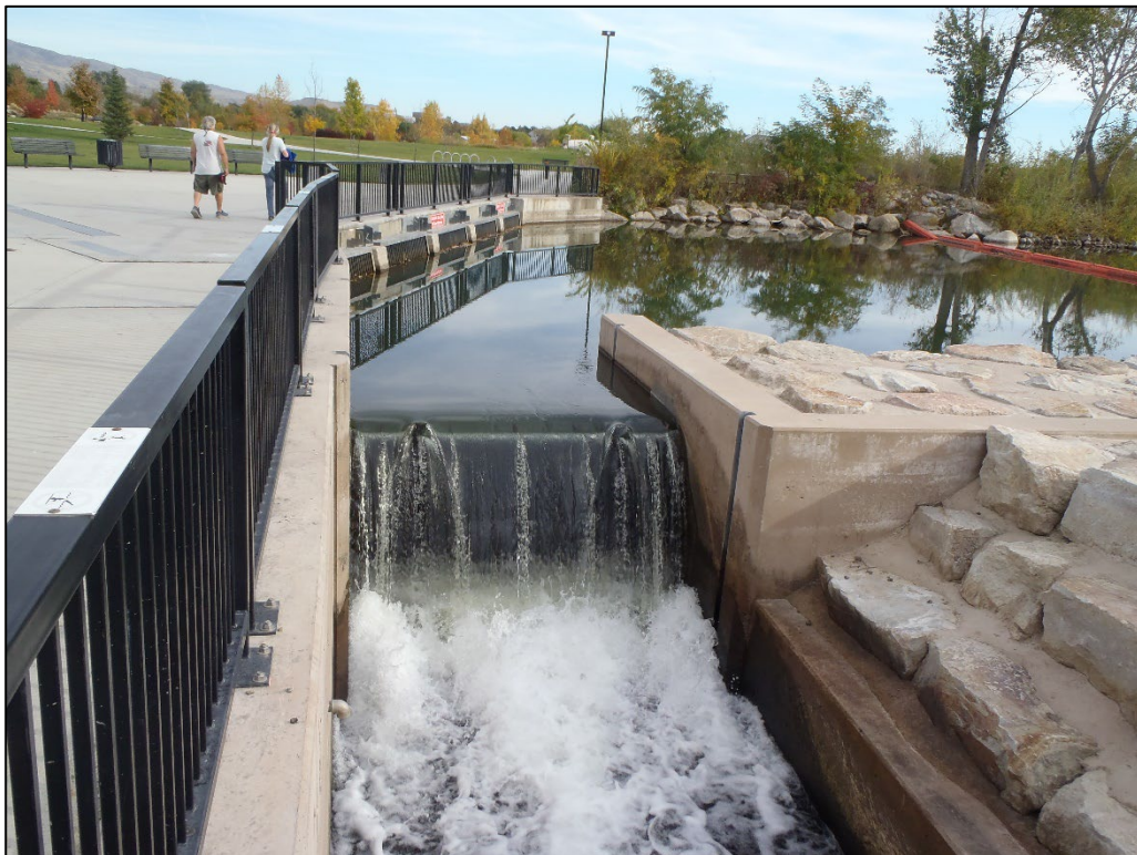
Photograph 6. Drop Structure 1 Sluiceway looking Upstream (October 2023).
