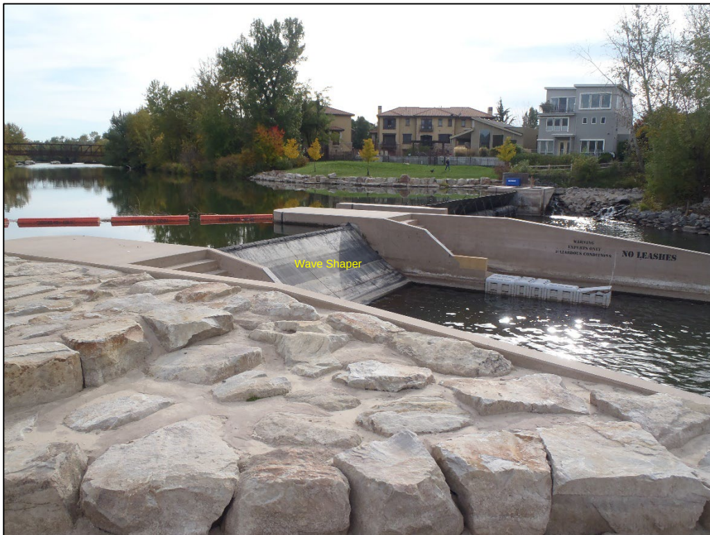
Photograph 5. Drop Structure 1 Wave Shaper looking Upstream (October 2023).
