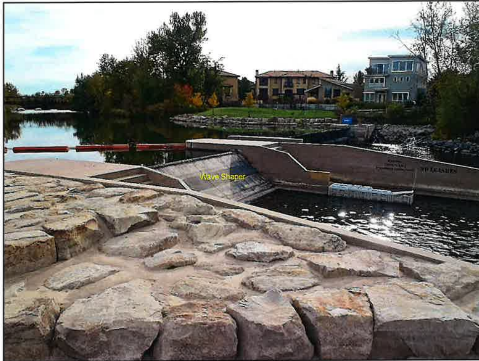
Photograph 5. Drop Structure 1 Wave Shaper looking Upstream (October 2023).
