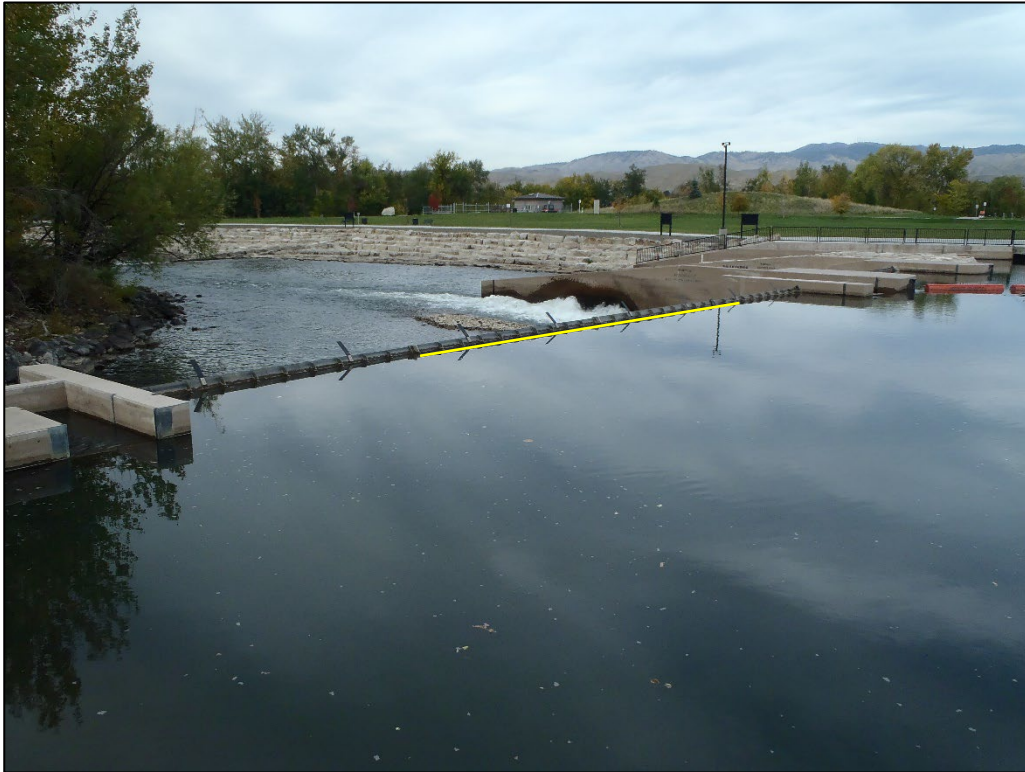
Photograph 1. Drop Structure 1 Gates 5 & 6 looking Downstream (October 2023).
