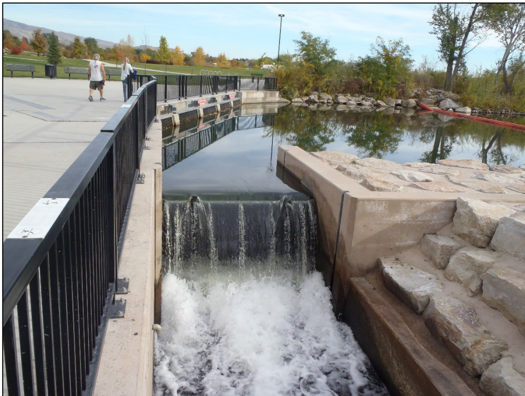
Photograph 6. Drop Structure 1 Sluiceway looking Upstream (October 2023).
