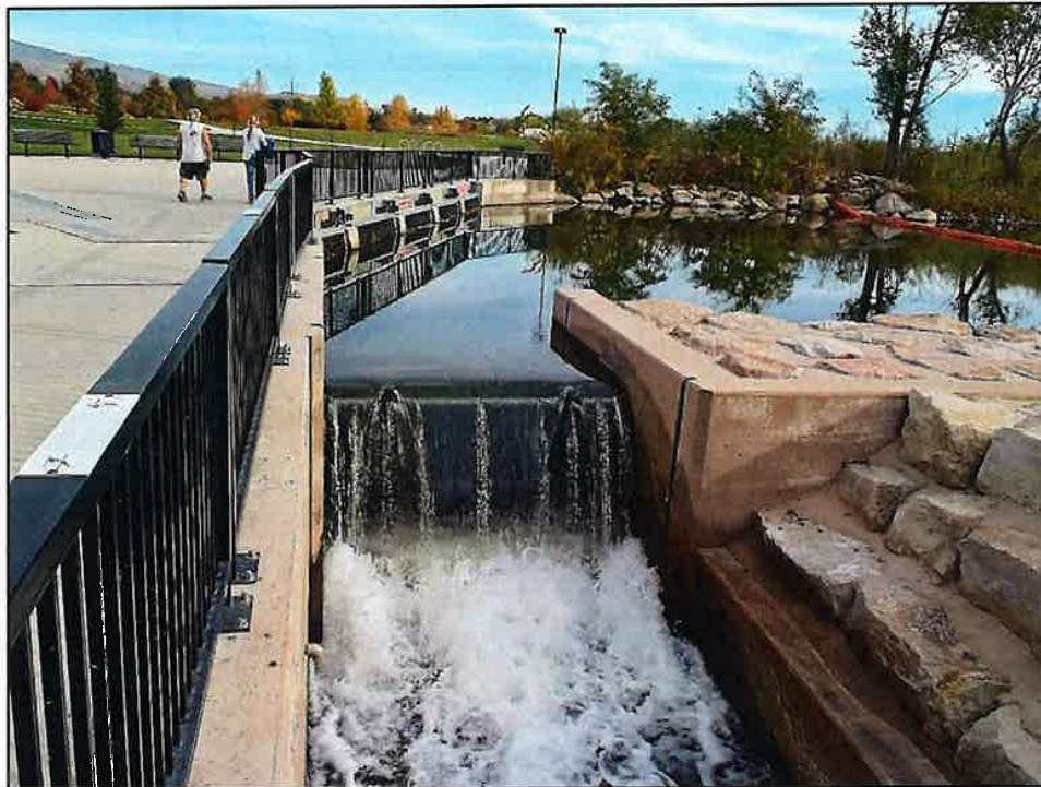
Photograph 6. Drop Structure 1 Sluiceway looking Upstream (October 2023).
